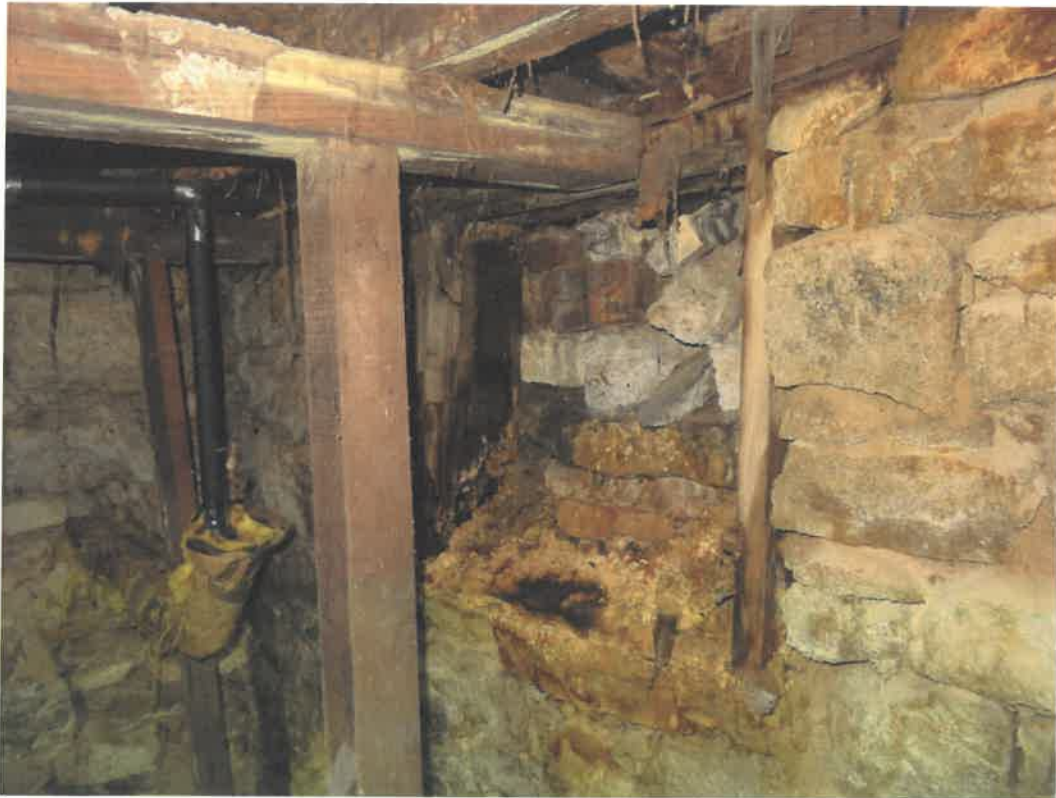
Photo 87 Building No. 37 – Flanigan’s/Rachelle Images (151 S 3rd St) Limestone Rubble Filled-In Coal Chute in Basement
