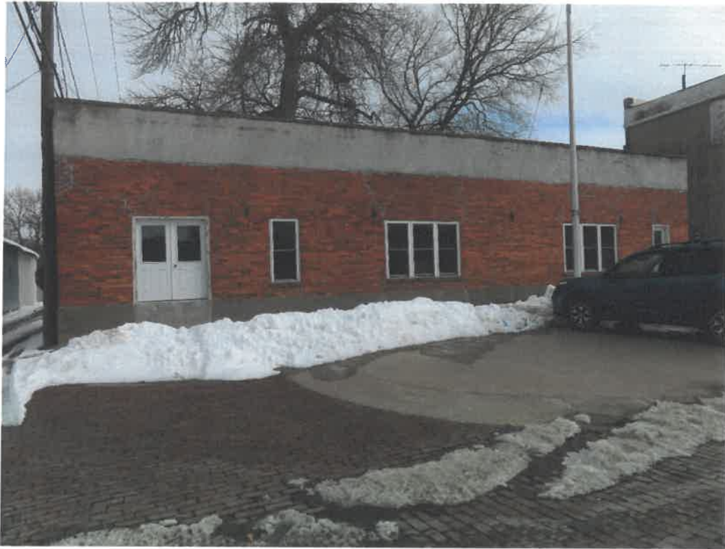
Photo 65 Building No. 27 – Keith Shuey Building (130 N 3rd St) Frontage Looking East
