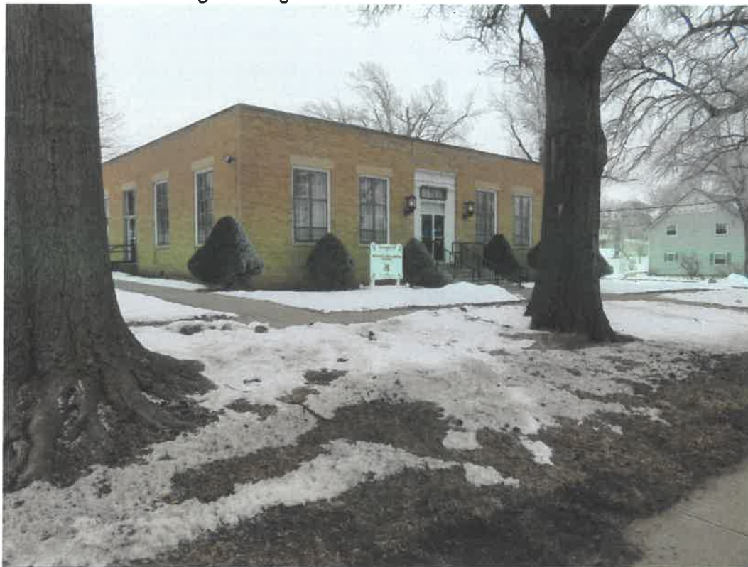
Photo 8 Building No. 8 – Tecumseh Post Office (484 Broadway St) Frontage Looking Northeast
