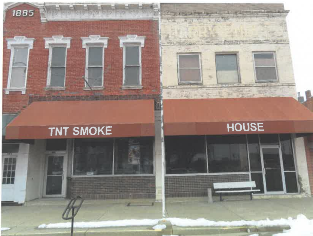
Photo 37 Building No. 20 – TNT Smoke House (366 Broadway St) Frontage Looking North
