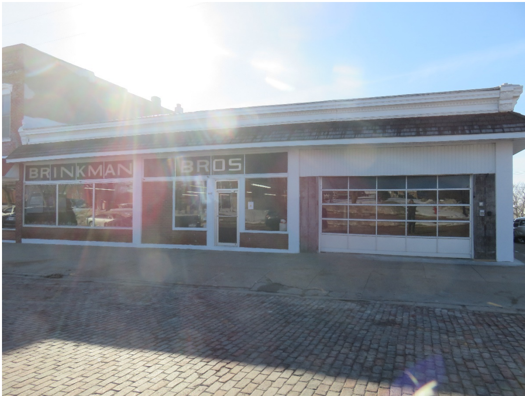
Photo 143 Building No. 56 – Brinkman’s Chevrolet & Buick (301/305/306 Clay St) Frontage Looking South
