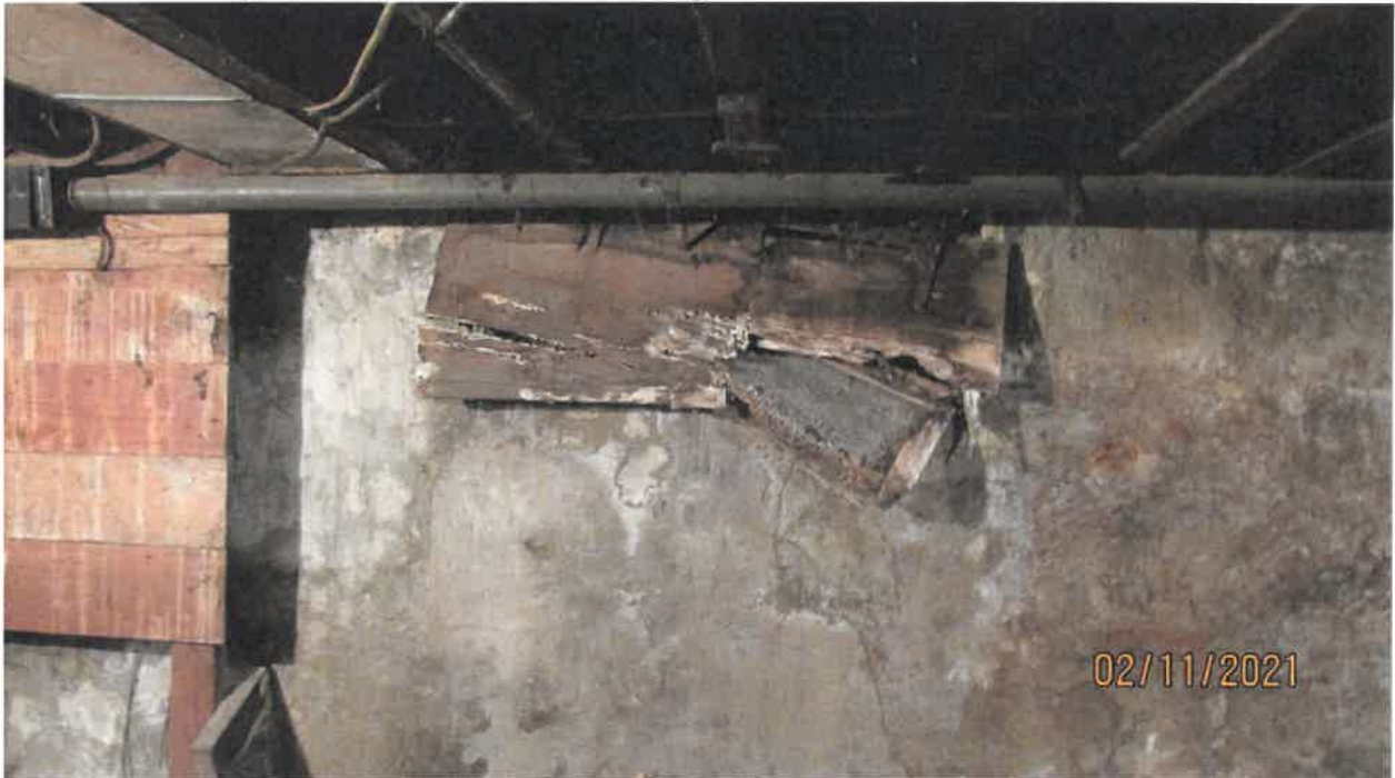
Photo 115 Building No. 45 – Hair by Luann (195 S 3 rd St) Open Vent on South Face of Building in Basement
