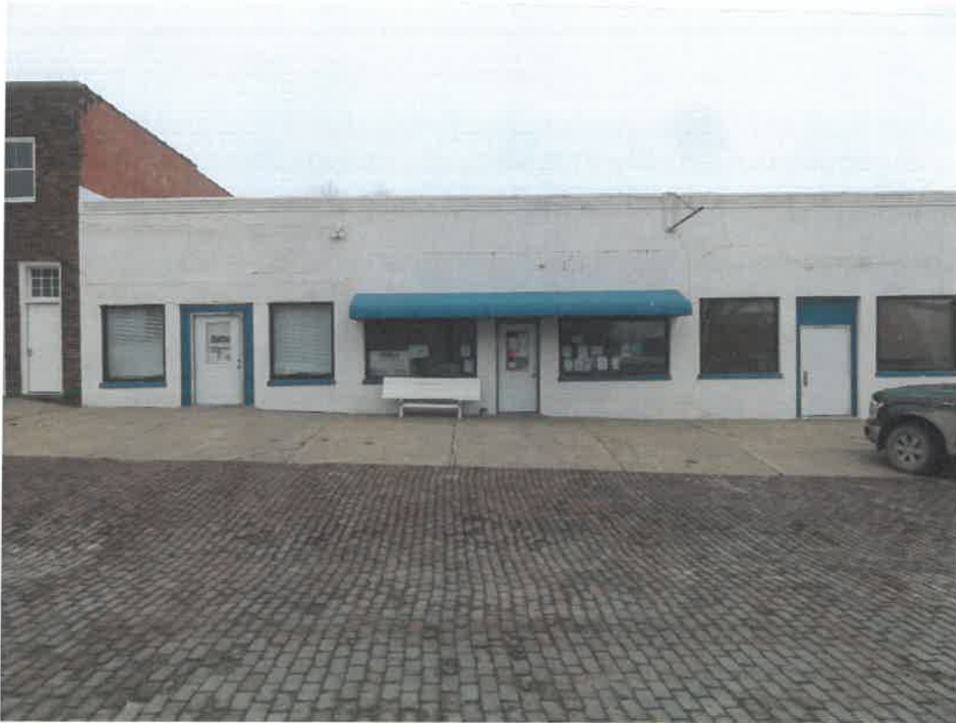
Photo 3 Building No. 3 – Senca Community Action (172 S 4th St) Frontage Looking East
