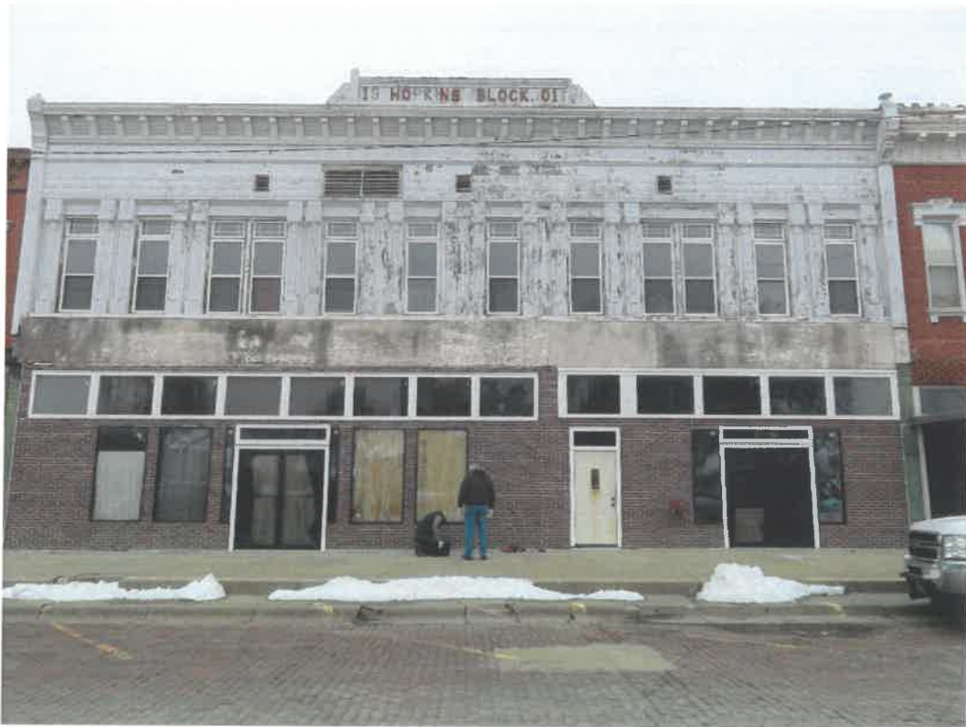
Photo 45 Building No. 22 – Hopkins Block (340 Broadway St) Frontage Looking North
