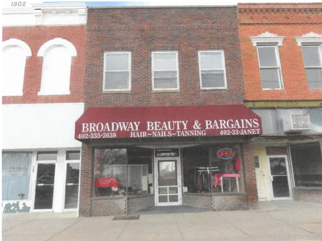
Photo 54 Building No. 24 – Broadway Beauty & Bargains (318 Broadway St) Frontage Looking North
