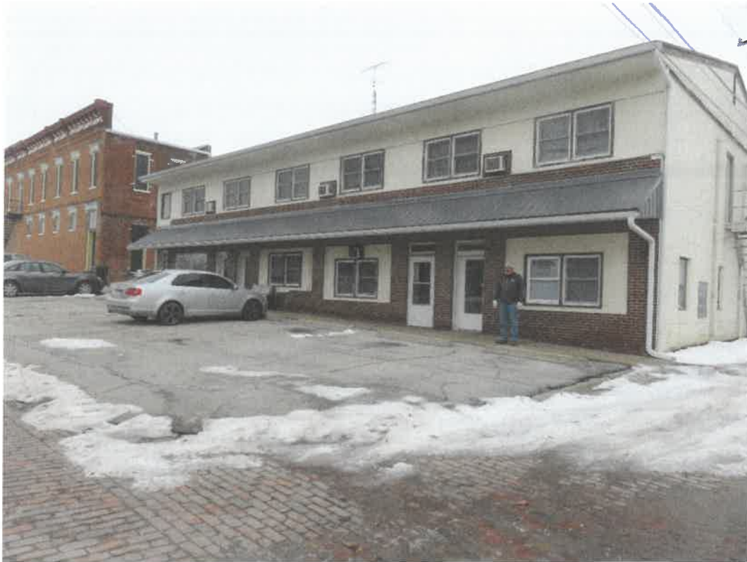
Photo 17 Building No. 16 – Town Square Apts./3 Other Businesses (131 N 4th St) Frontage Looking Southwest
