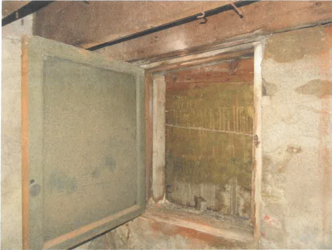
Photo 89 Building No. 38 – Ramsey Family Fountain (155 S 3rd St) Wood Plank/Concrete Filled-In Coal Chute in Basement
