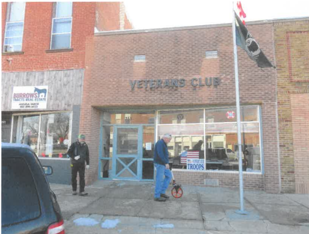
Photo 132 Building No. 53 – Veterans Club (255 Clay St) Frontage Looking South
