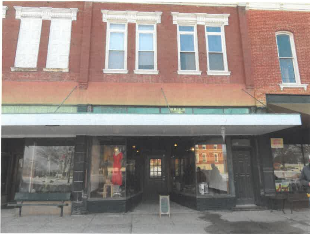
Photo 92 Building No. 39 – Remedy (171 S 3rd St) Frontage Looking West
