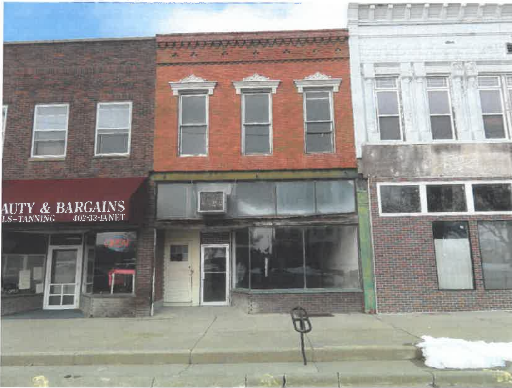
Photo 51 Building No. 23 – Steve Young Building (334 Broadway St) Frontage Looking North
