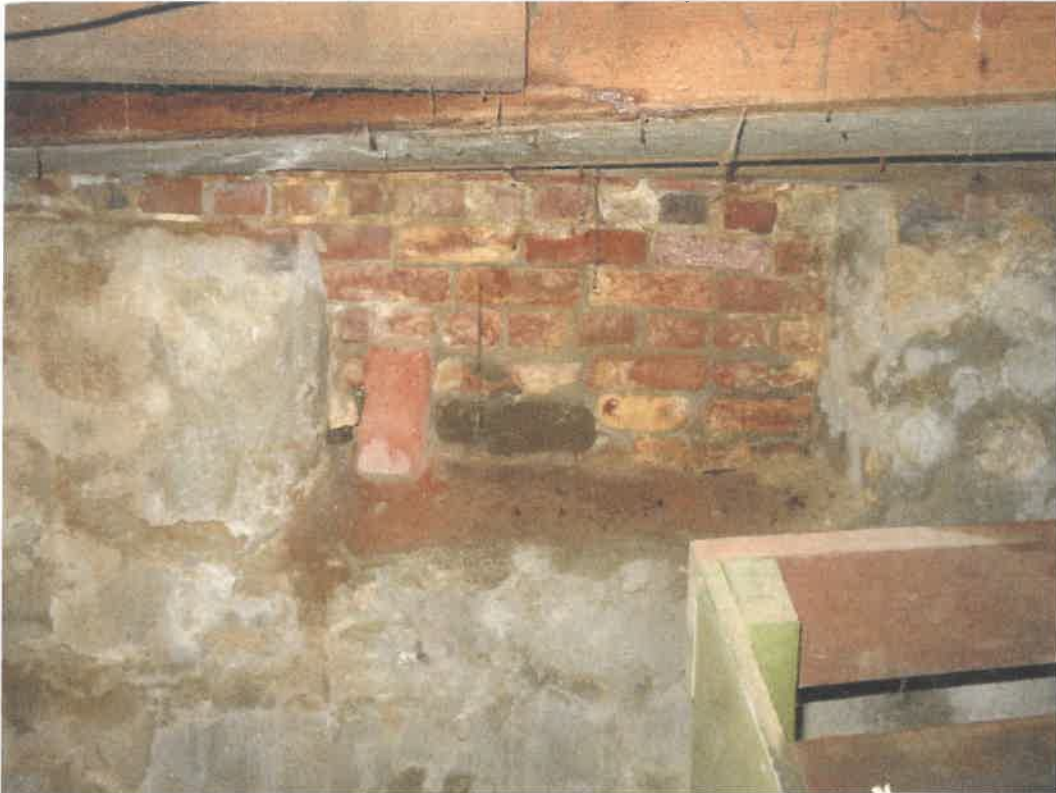
Photo 131 Building No. 52 – Bob Gregory Building (241 Clay St) Brick Filled-In Coal Chute in Basement
