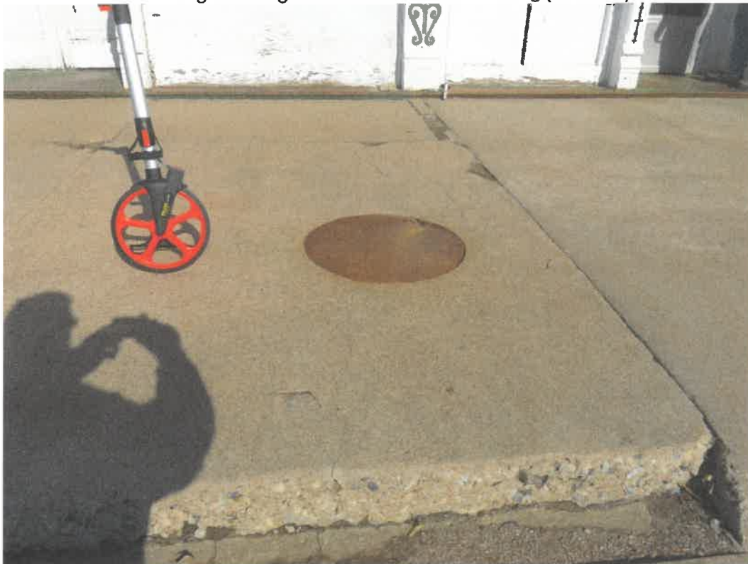
Photo 122 Building No. 47 – Hupka Farm Toys (266 Clay St) Manhole to Vault Under Sidewalk
