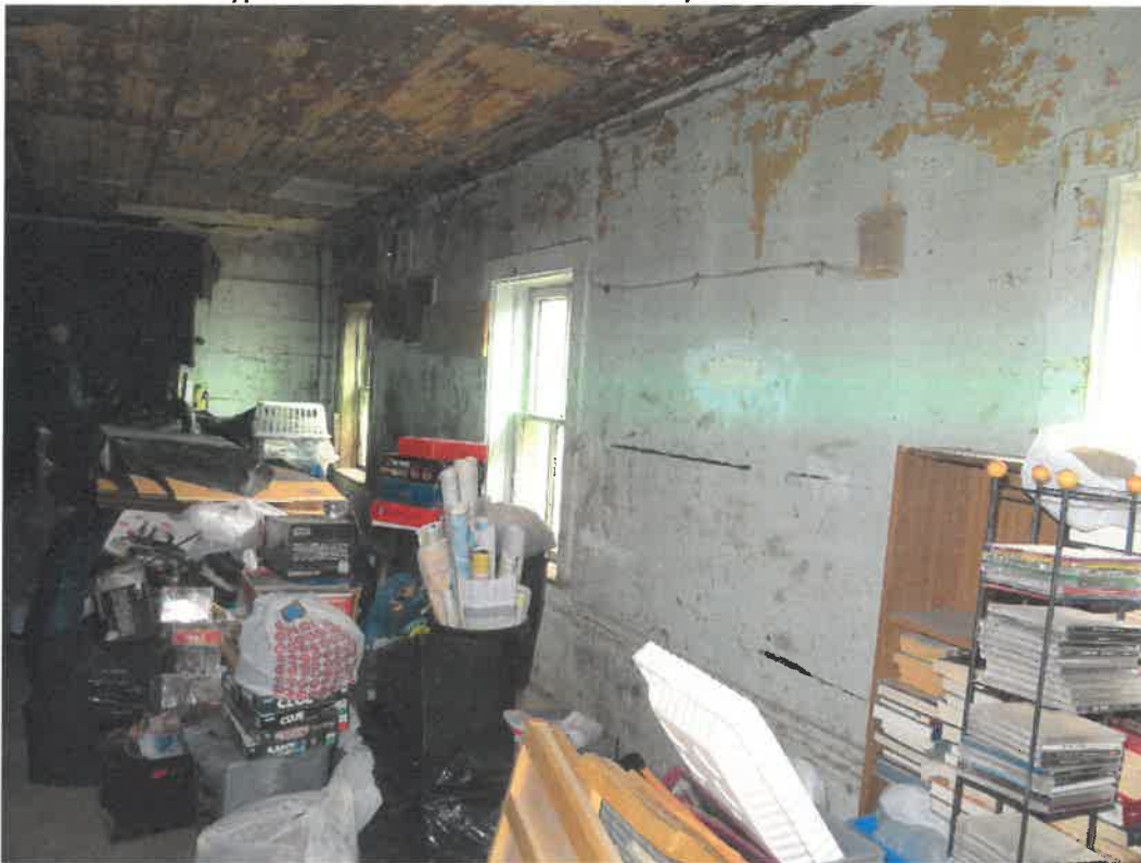
Photo 28 Building No. 17 – Nester & Mercure Attorneys (398 Broadway St) Typical Windows Looking into Basement Hall
