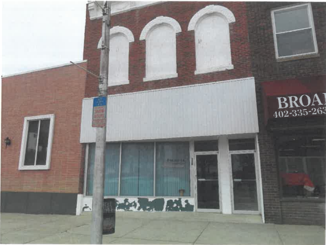
Photo 57 Building No. 25 – American National Bank – East Annex (310 Broadway St) Frontage Looking North
