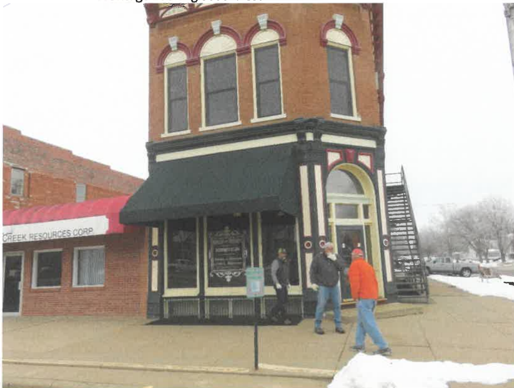
Photo 18 Building No. 17 – Nester & Mercure Attorneys (398 Broadway St) Frontage Looking North
