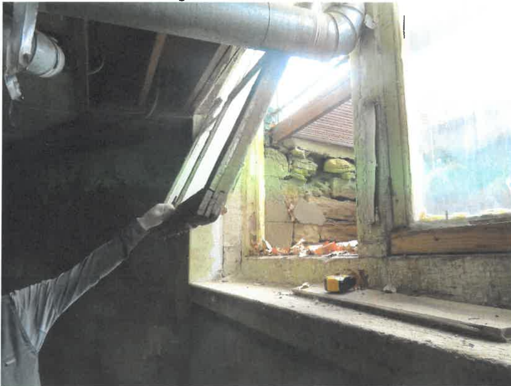
Photo 22 Building No. 17 – Nester & Mercure Attorneys (398 Broadway St) East End of Lightwell
