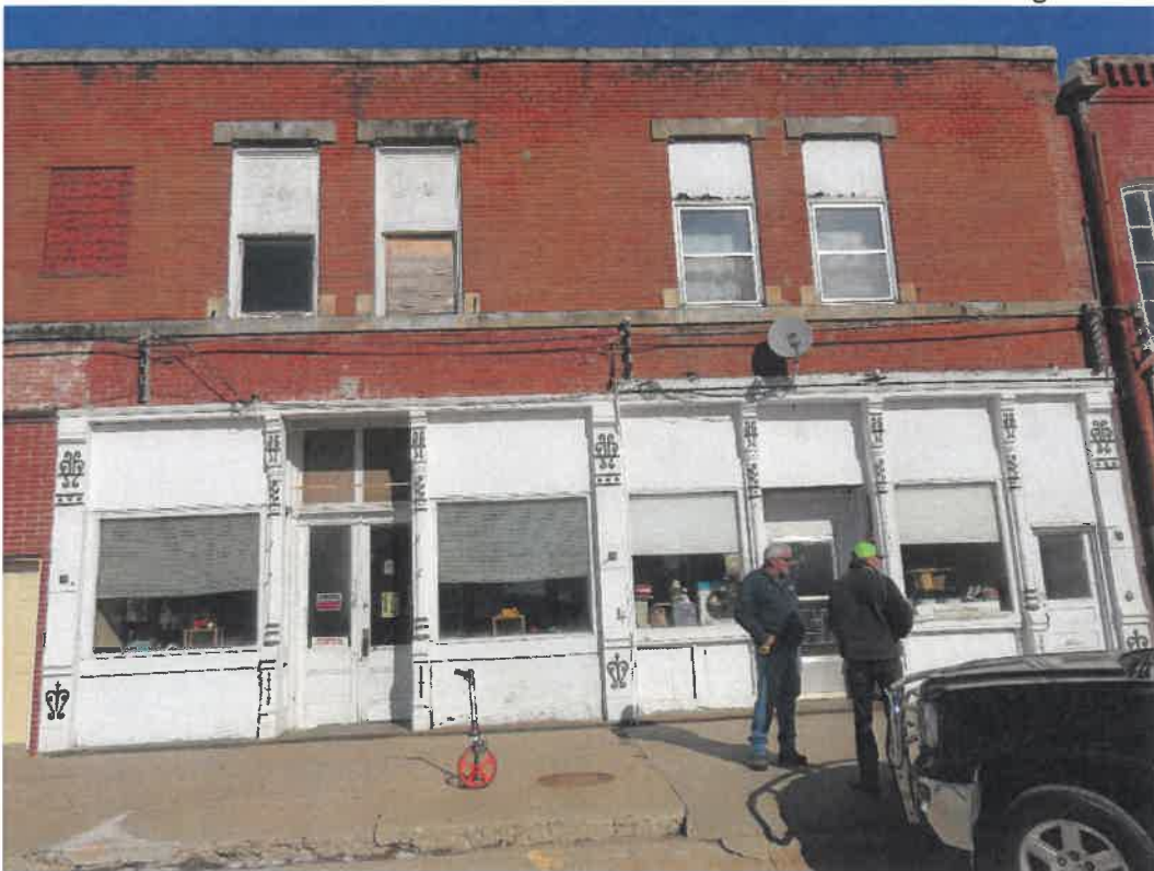
Photo 118 Building No. 46 – Blessing Heating & Plumbing (274 Clay St) Frontage Looking North – East Half of Building (Right Side)
