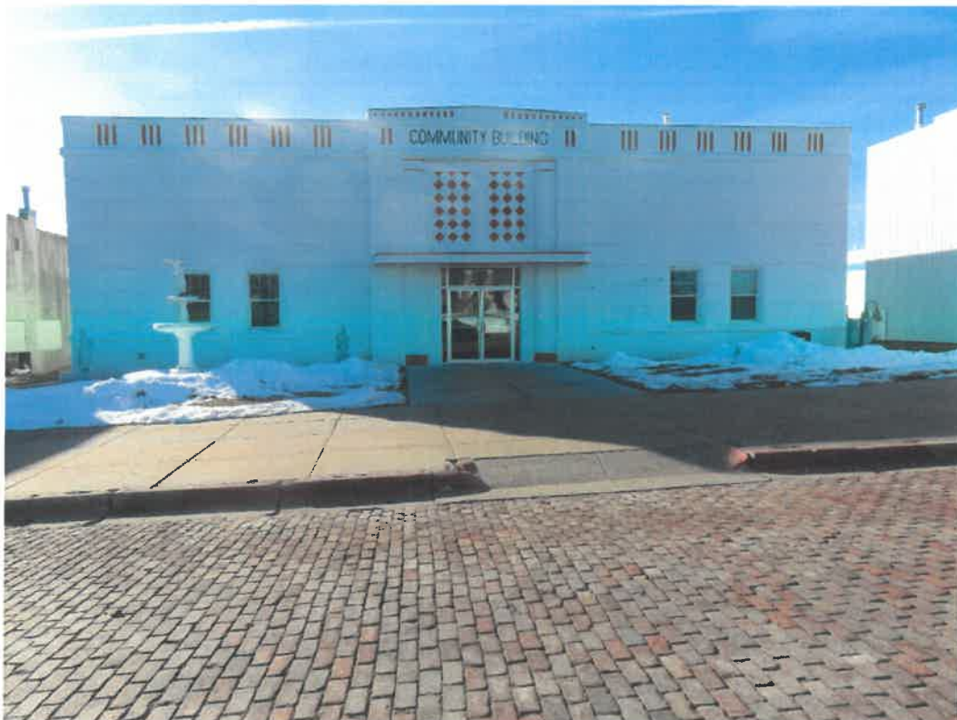
Photo 152 Building No. 58 – Tecumseh Community Hall (355 Clay St) Frontage Looking South
