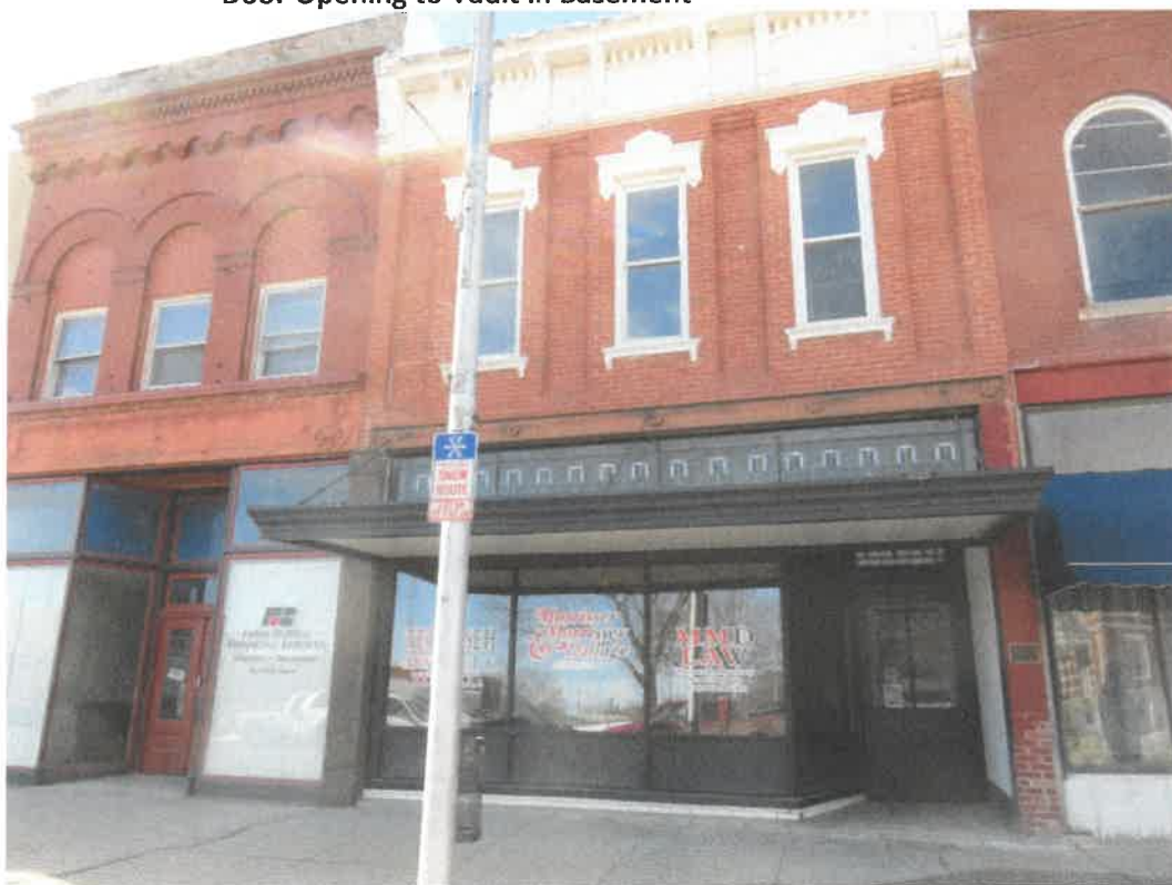
Photo 100 Building No. 42 – Morrissey, Morrissey & Dalluge (177 S 3rd St) Frontage Looking West
