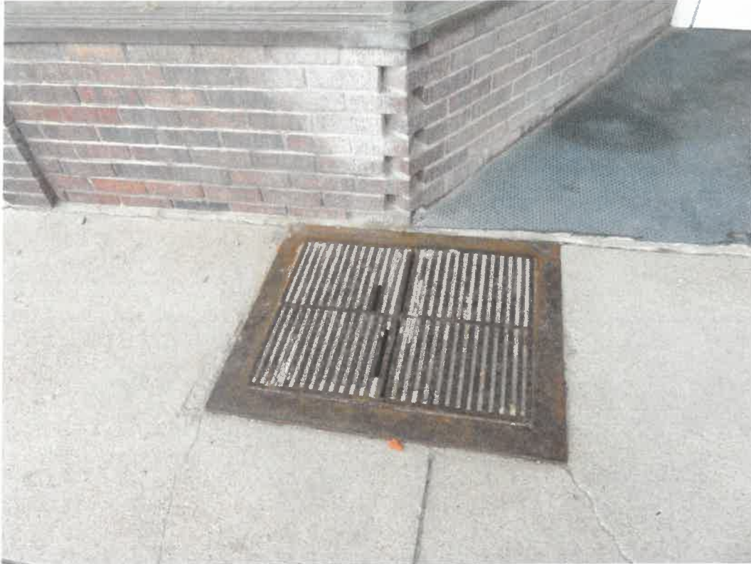
Photo 55 Building No. 24 – Broadway Beauty & Bargains (318 Broadway St) Partially Filled-In Coal Chute in Sidewalk
