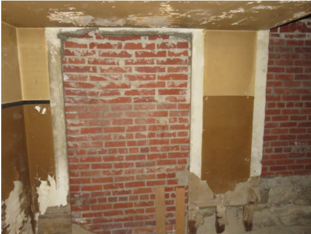
Photo 61 Building No. 26 – American National Bank (306/310 Broadway St) Brick Filled-In Vault at East End of South Wall in Basement
