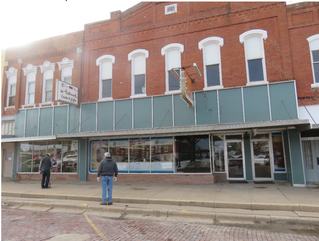
Photo 76 Building No. 34 – Chief Rexall Drugs (123/125 S 3rd St) Frontage Looking West
