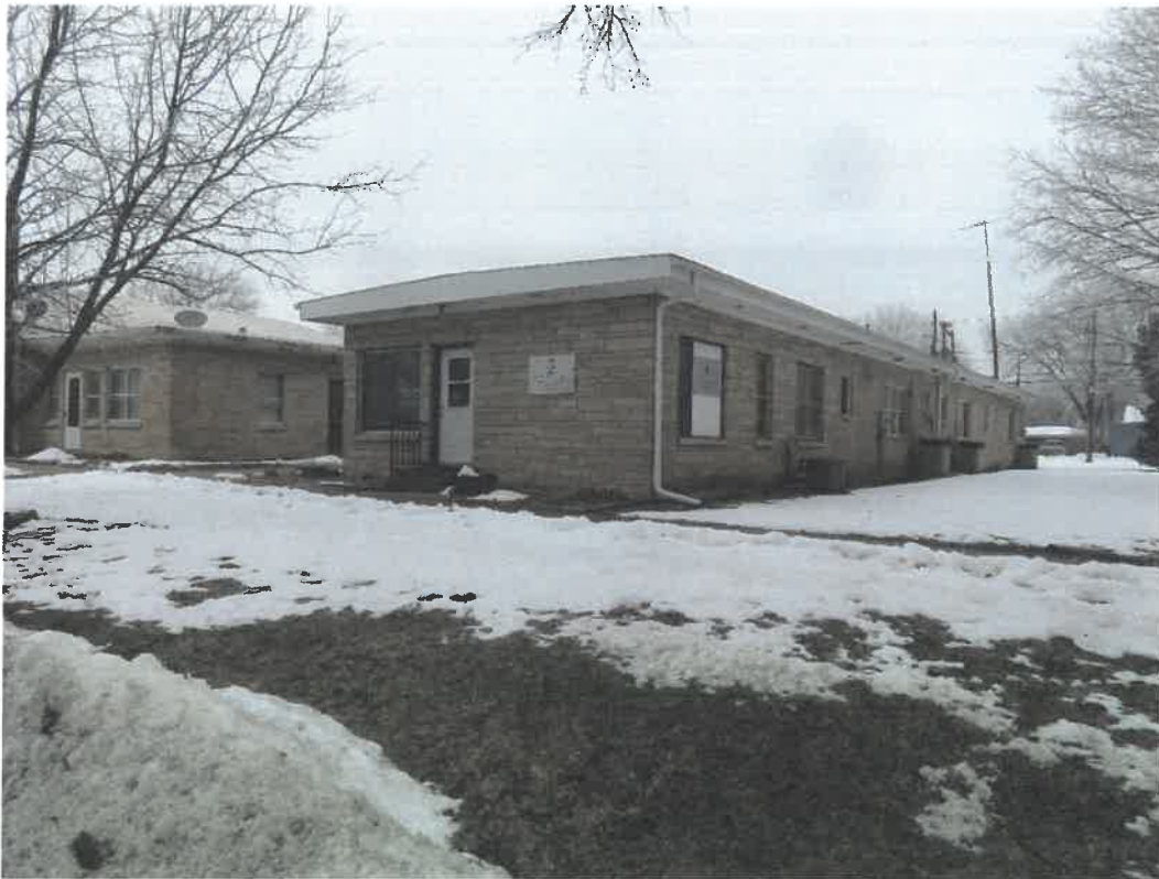
Photo 9 Building No. 9 – Richard R. Smith Law Office (454 Broadway St) Frontage Looking Northwest
