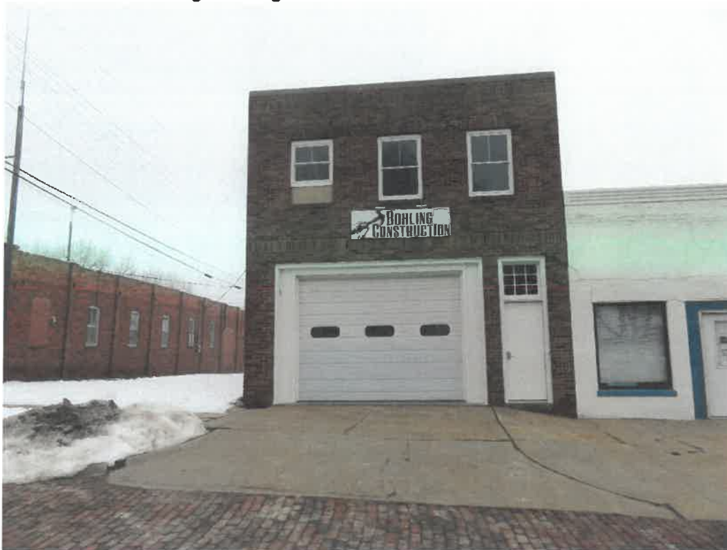
Photo 4 Building No. 4 – Bohling Construction (160 S 4th St) Frontage Looking East
