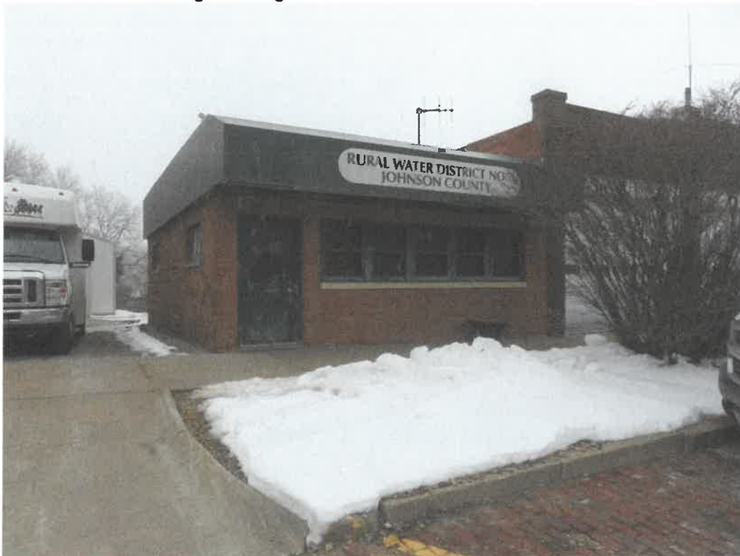
Photo 6 Building No. 6 – Johnson County Rural Water District (134 S 4th St) Frontage Looking East
