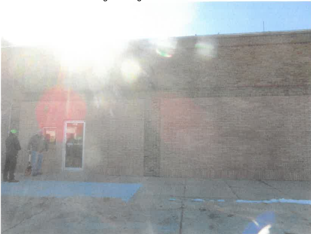
Photo 130 Building No. 52 – Bob Gregory Building (241 Clay St) Frontage Looking South
