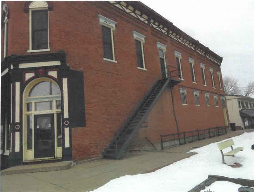
Photo 19 Building No. 17 – Nester & Mercure Attorneys (398 Broadway St) Frontage Looking Northwest
