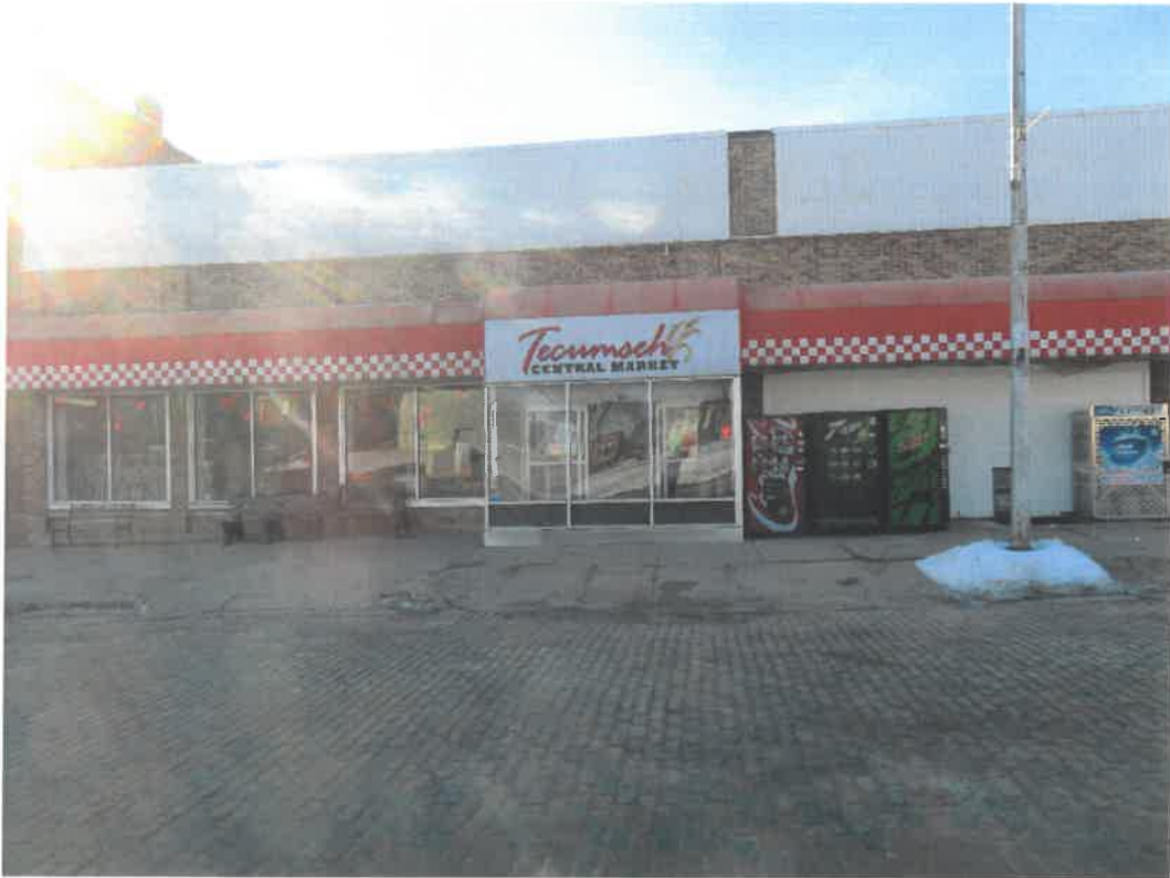
Photo 153 Building No. 59 – Tecumseh Central Market (381 Clay St) Frontage Looking South
