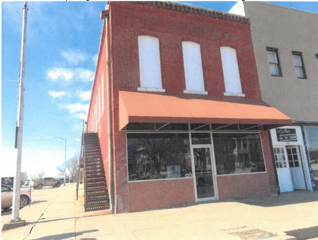
Photo 110 Building No. 45 – Hair by Luann (195 S 3rd St) Frontage Looking West
