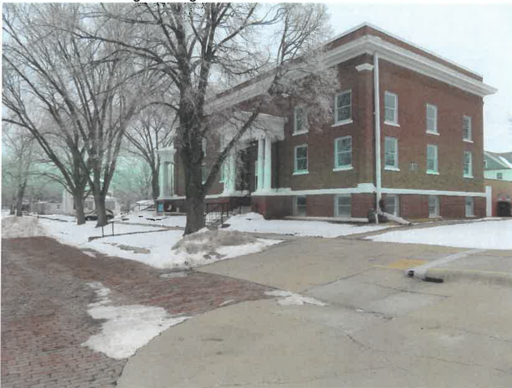
Photo 16 Building No. 15 – Methodist Church (190 N 4th St) Frontage Looking Northeast
