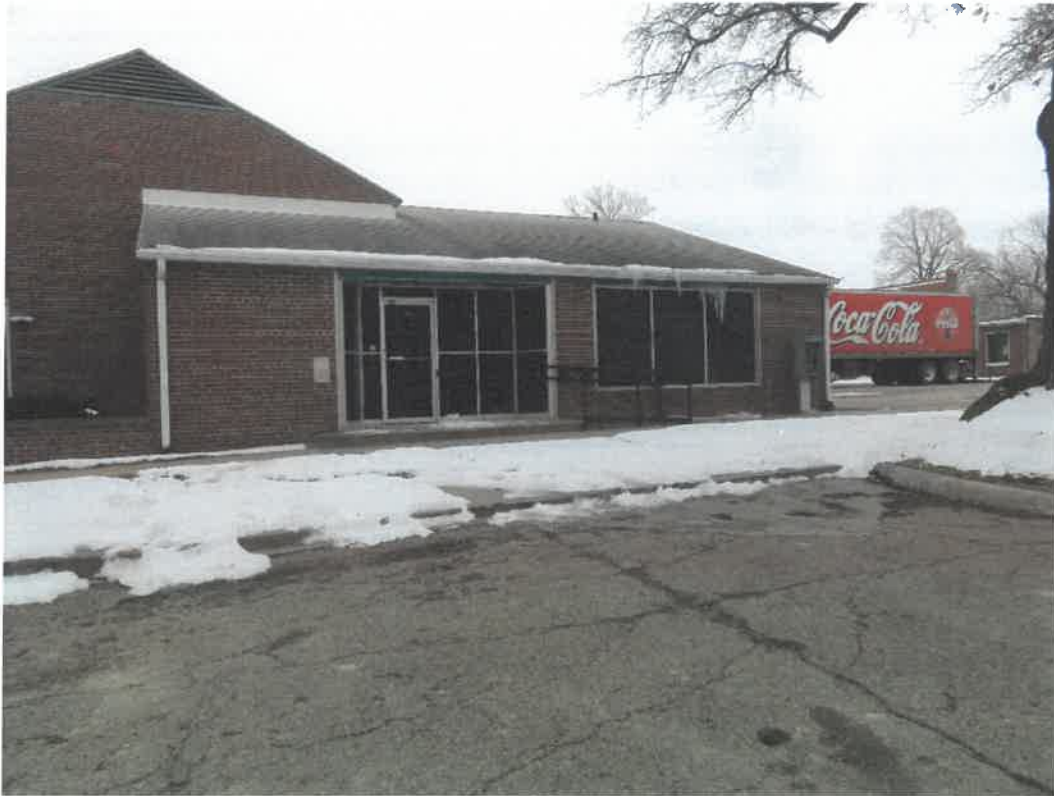
Photo 13 Building No. 13 – Fire Rivers RC&D (140 N 4th St) South Side of Frontage Looking East
