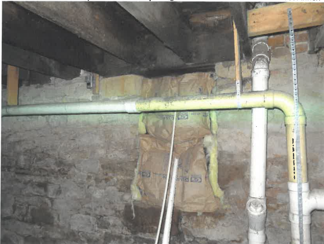
Photo 160 Building No. 59 – Tecumseh Central Market – East Annex (381 Clay St) Typical Partially Filled-In Window Opening in Basement on East Side of East Annex
