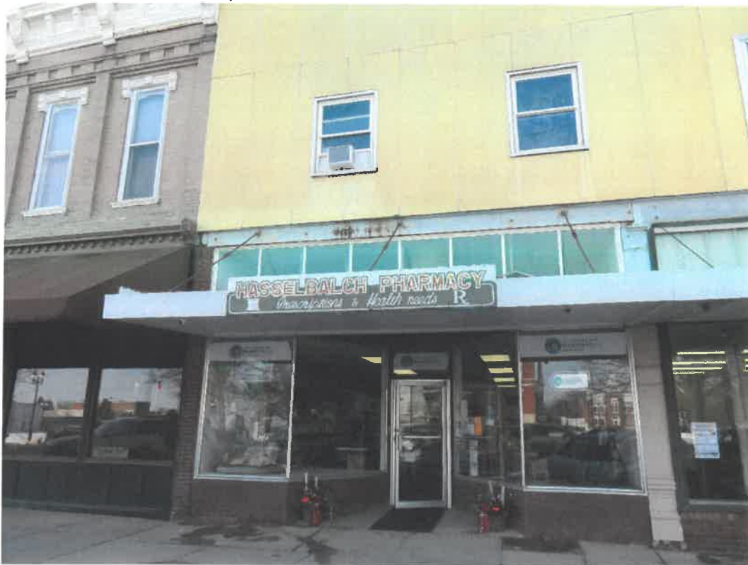
Photo 82 Building No. 36 – Hasselbach Pharmacy (143 S 3rd St) Frontage Looking West
