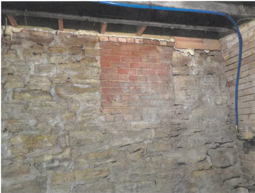
Photo 142 Building No. 55 – Johnson County Museum (235 S 3rd St) Brick Filled-In Coal Chute on North Wall of West Annex in Basement
