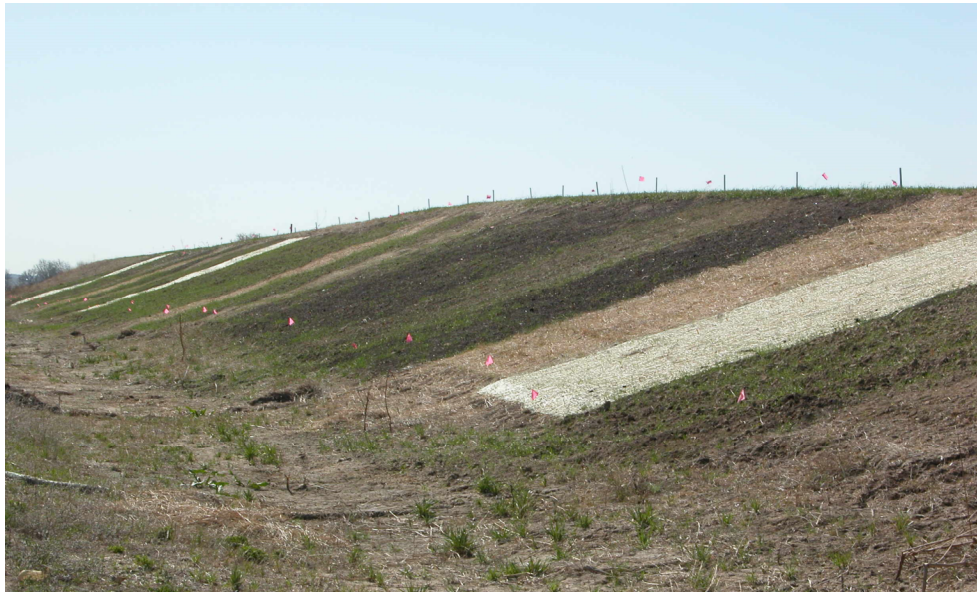
NDOT research plots along a highway
