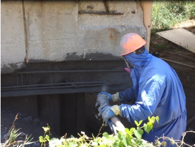
Figure 7.31—Concrete Patching at Abutment with Shotcrete
