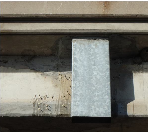
Figure 7.41—Crack Epoxy Injection on S070 10755
