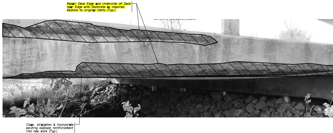
Figure 7.36—Note on Plan for Requiring Use of Shotcrete (example taken from S275 03181, CN 32267, 2016)
