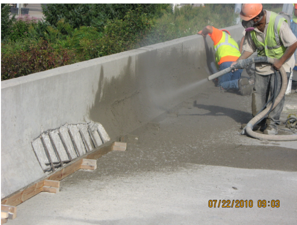
Figure 7.33—Concrete Patching at Bridge Rail, with Shotcrete
