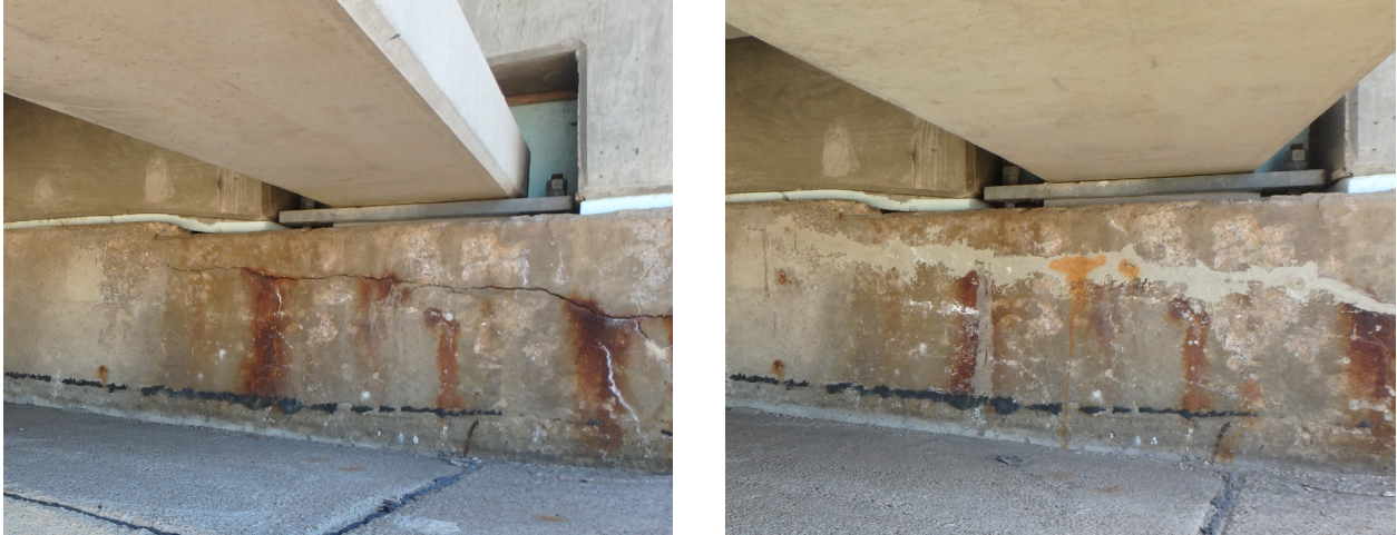
Figure 7.38—Epoxy Crack Injection (Before on the Left, and After on the Right)
