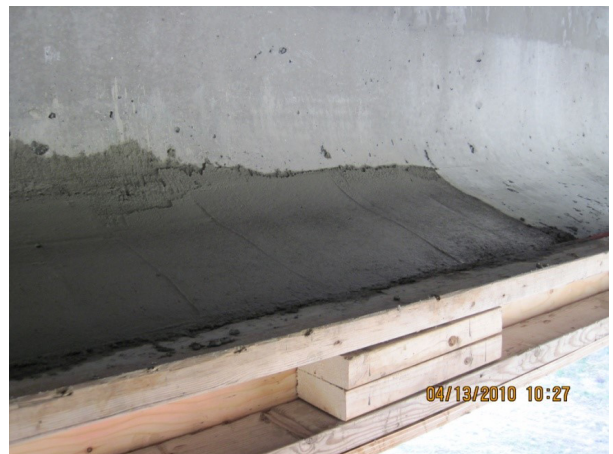
F. Finished Grout
