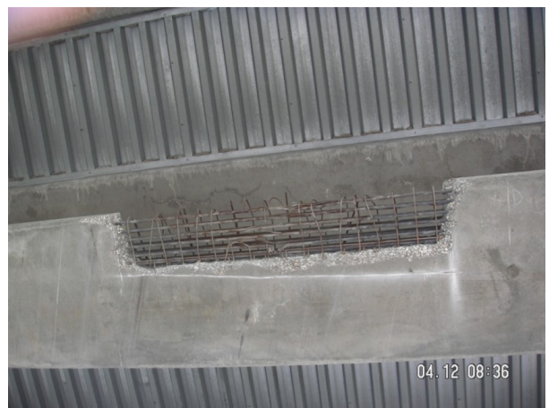
B. Concrete Removal
