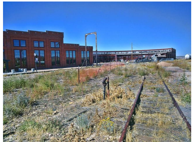
Historical railroad roundhouse and maintenance yard.
