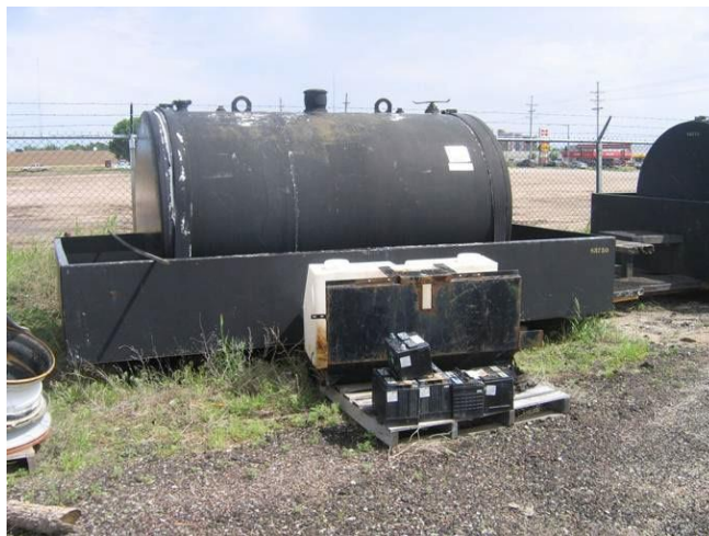
Old batteries stored outside and exposed to the elements. Also, AST with secondary containment.
