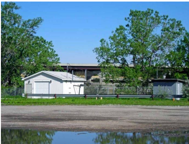
Typical groundwater remediation sheds.
