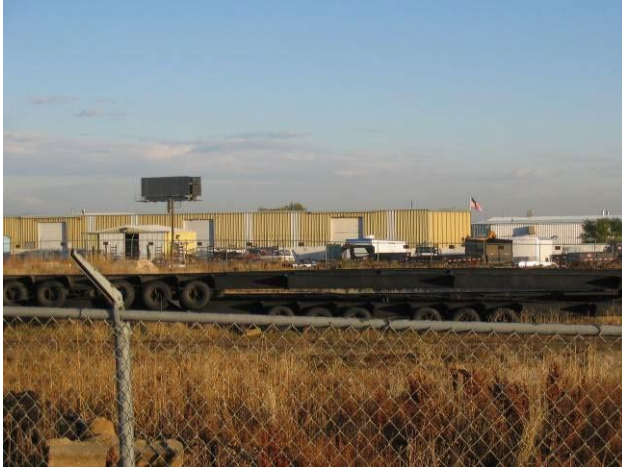
Vehicle bays adjacent to highway right-of-way.
