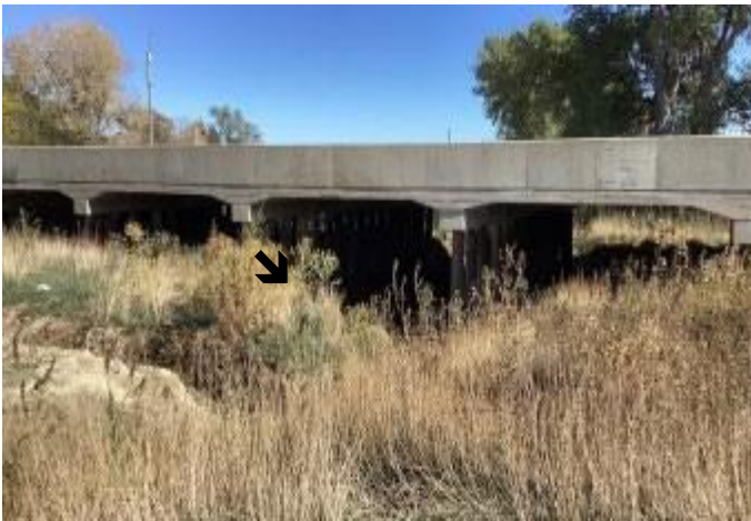
Profile of a bridge during inspection.
