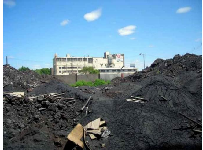
Ash waste stockpiles at a steel foundry. Litter and some broken pallets are also strewn about.
