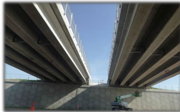
Kearney East Bypass
