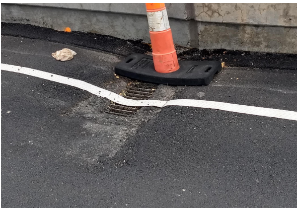
Figure 7.47—Drain in Driving Lane
