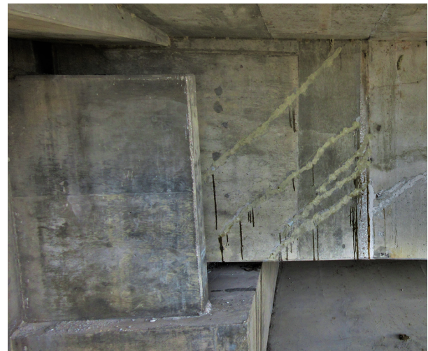
Figure 7.42—Crack Epoxy Injection on S002 50816
