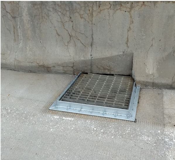
A. Shoulder Drain With Frame Prior to Overlay
