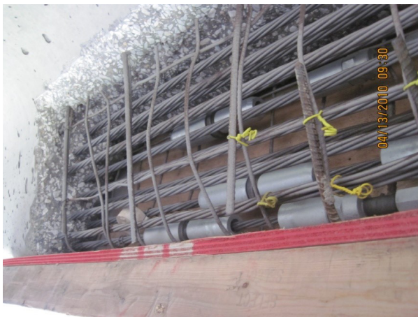
E. Splices Installed
