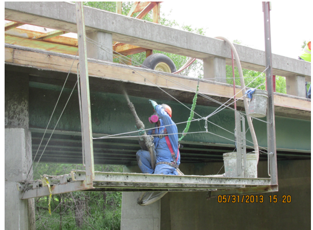
Figure 7.32—Concrete Patching at Deck Edges, with Shotcrete
