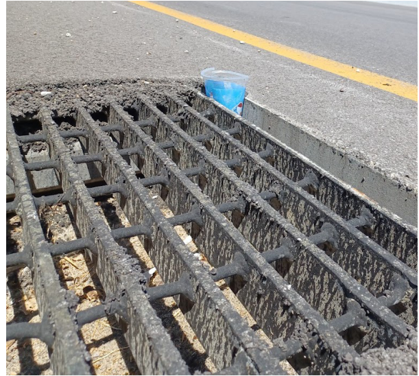
B. Shoulder Drain With Frame After Overlay
