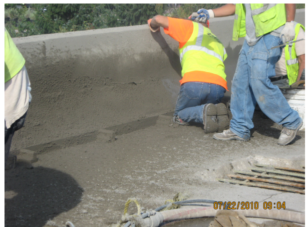
Figure 7.33—Concrete Patching at Bridge Rail, with Shotcrete
