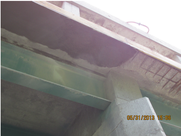
Figure 7.32—Concrete Patching at Deck Edges, with Shotcrete
