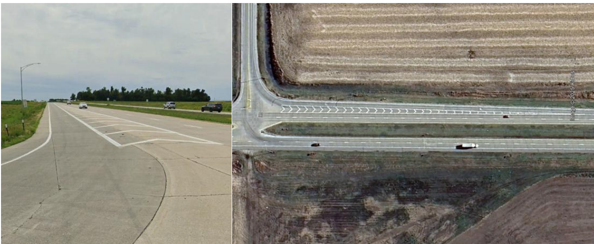
Example Right-Turn Lane Built by NDOT at Highway Junction
