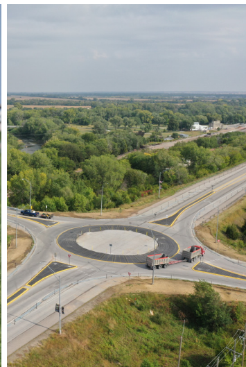
Roundabout on US-6 Near Ashland
