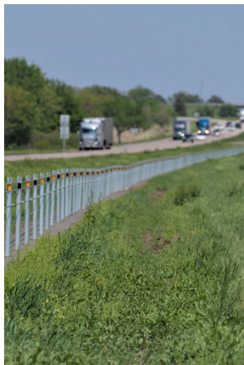
Cable Median Barrier on I-80
