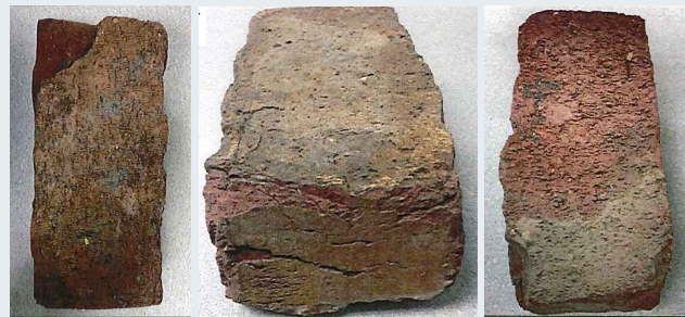
Damage on underside of bricks, not visible from surface
