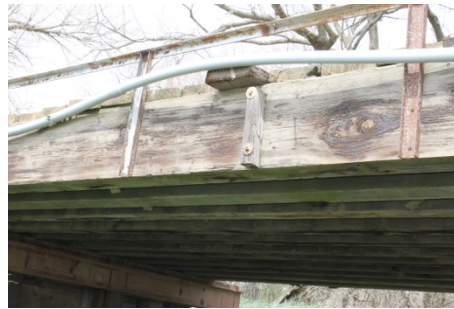
Fig. 21. View under the bridge
