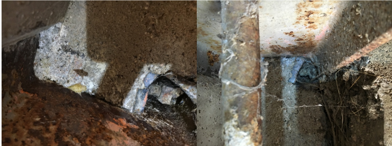
Fig. 46. Supporting conditions for girders
