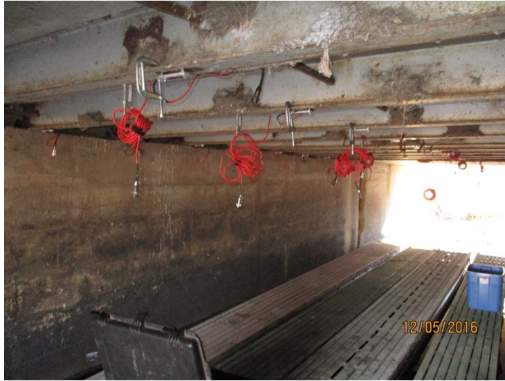
Fig. 47. Transducers attached to the bottom of girders
