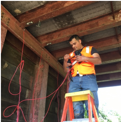
Fig. 2. Instrumentation of the bridge
