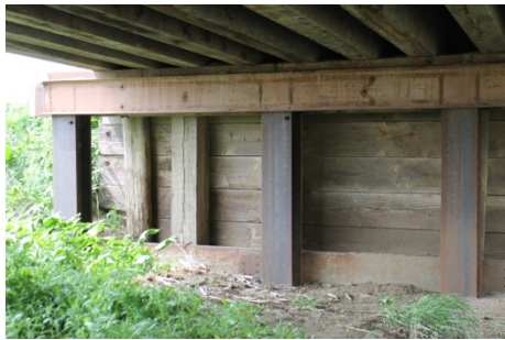
Fig. 20. New steel support
