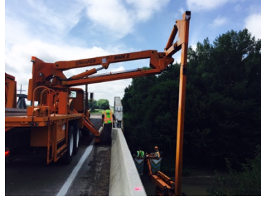
Fig. 5. Snooper operating on the bridge
