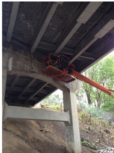
Fig. 3. Boom truck operating under the bridge
