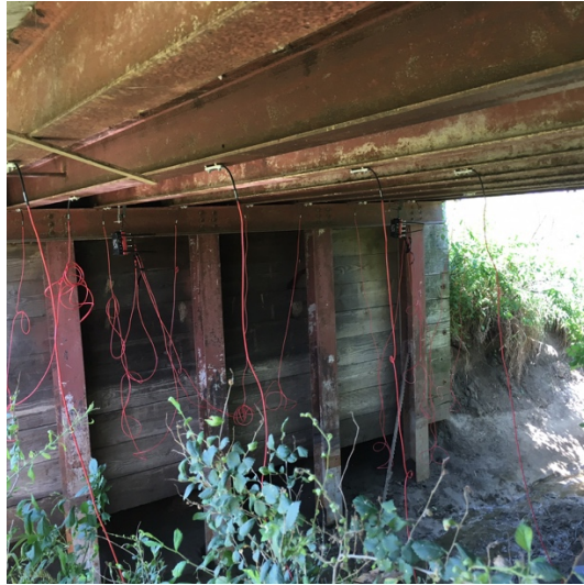
Fig. 14. Transducers attached to girders
