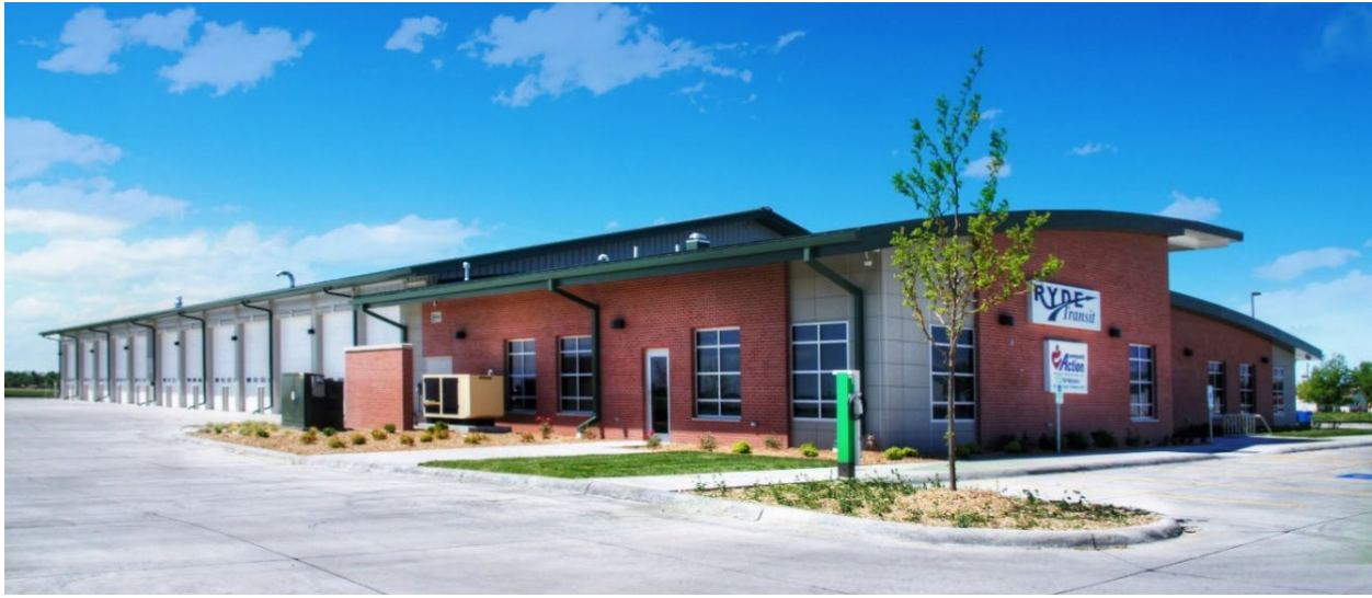
Figure 2. Nebraska Transit Assets, RYDE Transit Station
