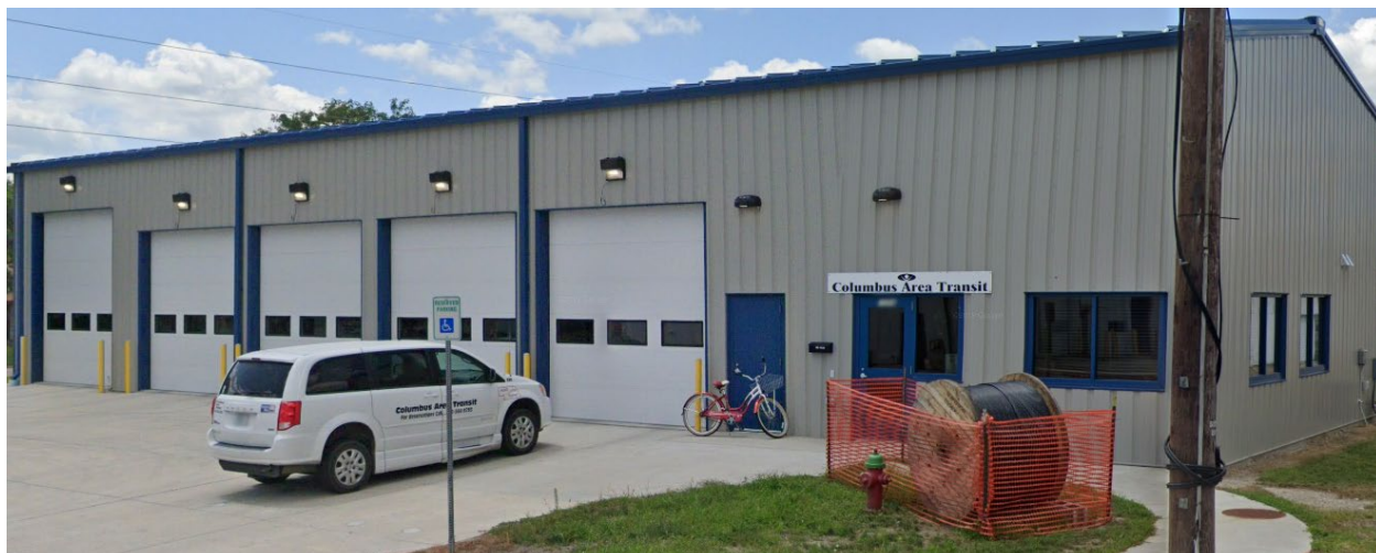
Figure 5. Columbus Area Transit Facility
